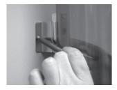
Mark location of wall mount bracket using mounting holes.
