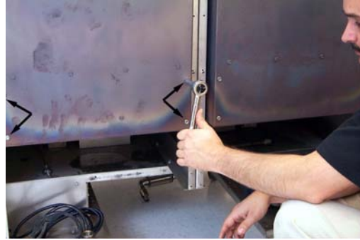
Removing bolts (arrows) securing flue to frypot.
