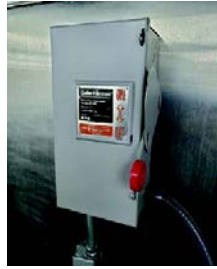
Combi-Duo Unit Independently Fused Power Supply Line
