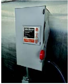
Single Unit Independently Fused Power Supply Line
