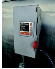
Combi-Duo Unit Independently Fused Power Supply Line
