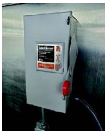
Single Unit Independently Fused Power Supply Line
