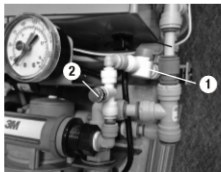
1 - blend line shutoff valve 2 - blending valve
