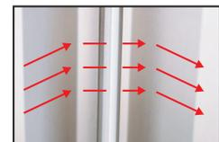
Formed side wall reduces 'drumming' vibration.
