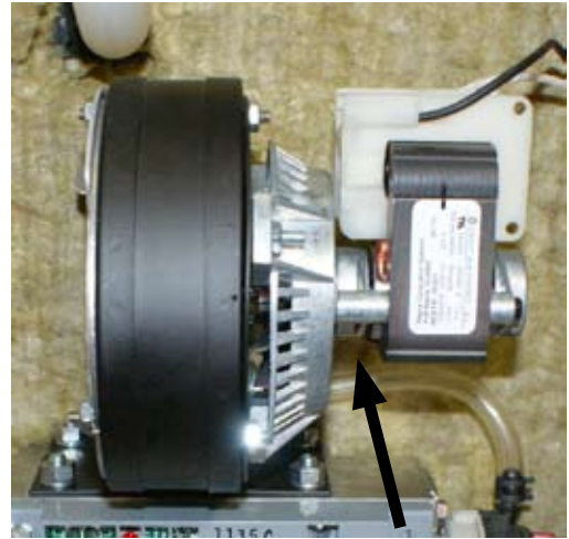
Fan Pressure Switch Hose
