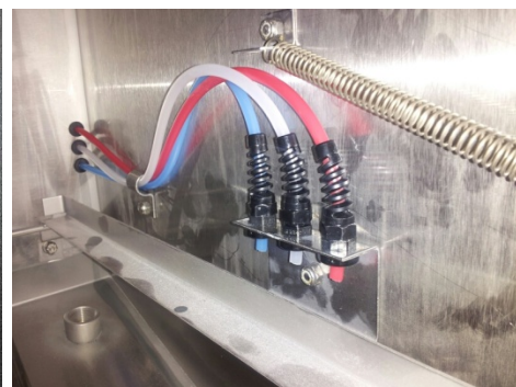
Chemical inlet tubes
