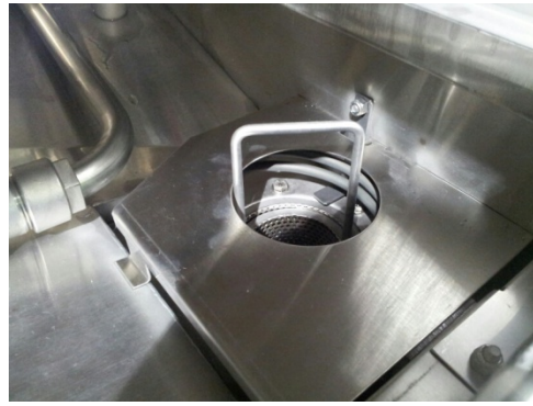
Placement of the pump filter into the drain sump
