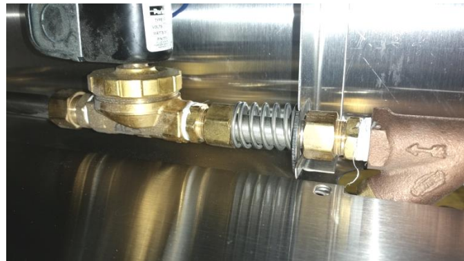
Showing 1/2" H2O solenoid, also stainless 1.5" drain tube
