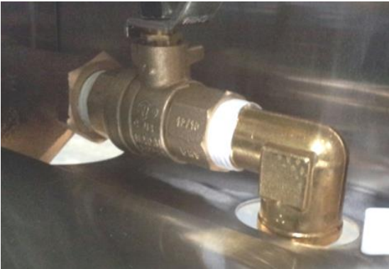
Drain hose connection to drain pipe
