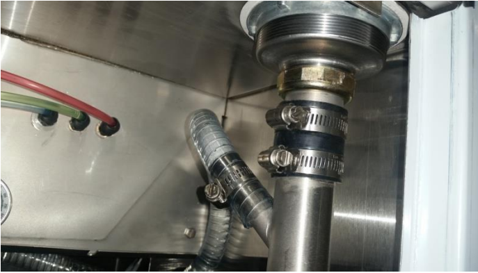
Drain hose connection to drain pipe
