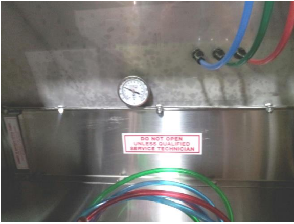
Showing chemical lines and temp gauge in cabinet
