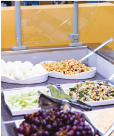
Bloomington Cold Mechanicals (BCM) utilize extra deep wells with recessed, adjustable rails so pans sit beneath the surface of the counter. This allows a blanket of cool air to float above the food, keeping the food fresher, longer.
