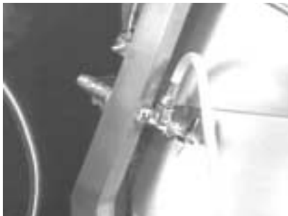
Use pipe dope to connect and tighten the water supply line (1/2" npt) to the connection at the rear of the unit.
