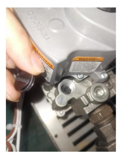
12. Keep turning until ring comes out and existing spring is exposed.
