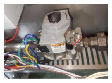
11. After cover is removed, use a small screwdriver to carefully turn counterclockwise, the plastic spring retainer ring shown below.
