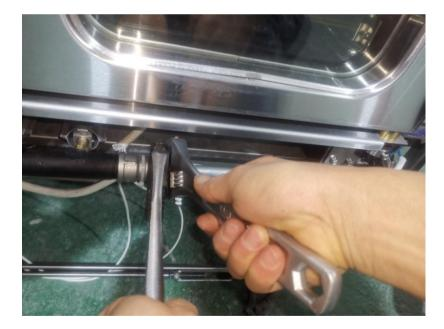
7. Loosen nuts holding manifold pipe to bracket and remove screws in front of manifold bracket holding it to oven frame. Cut cable ties holding electrical wires to manifold assembly (remember where they are so you can replace them with new cable ties during reinstallation.)
