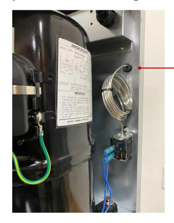
Run the sensing bulb out of the hole made and use the rubber grommet to seal the hole.
