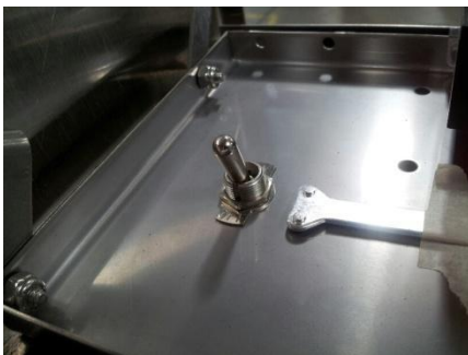
De-lime switch in control box
