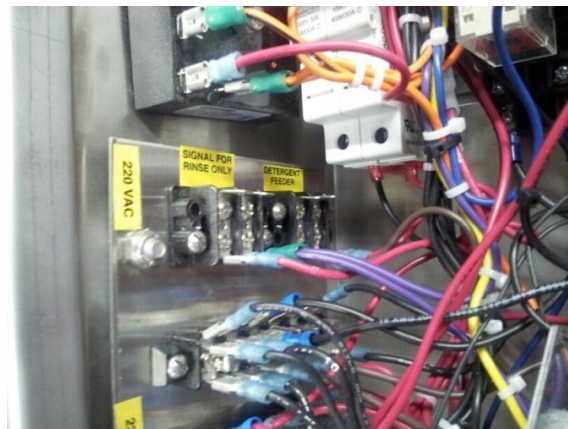
Showing dispenser signal connection terminals
