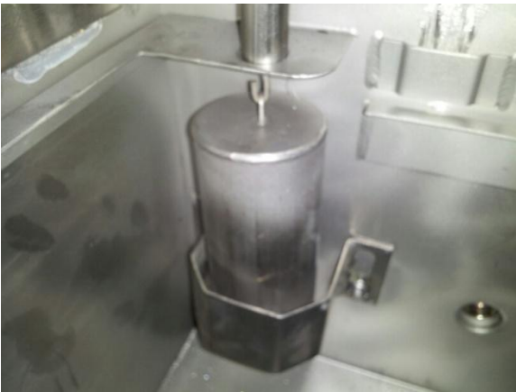
Wash tank float and tank overflow
