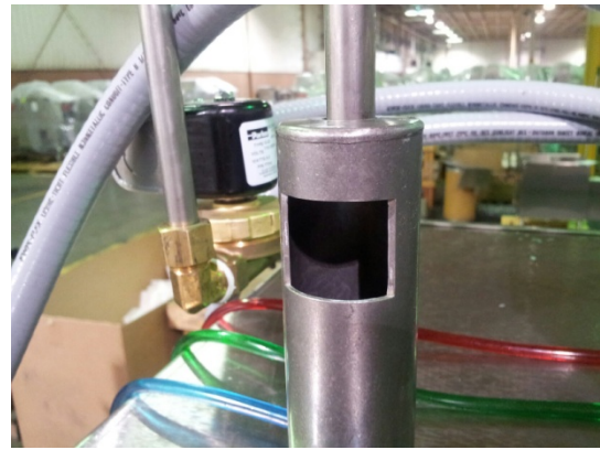
ASSE approved air gap (backflow preventer)
