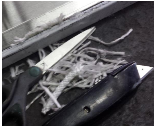
Figure 1 - After cutting existing door gasket
