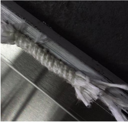
Figure 2 - Before cutting existing door gasket
