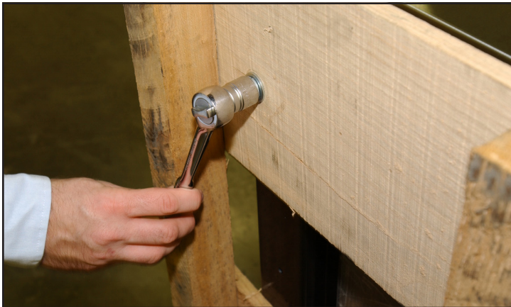
Removing skid from bottom of cabinet.
