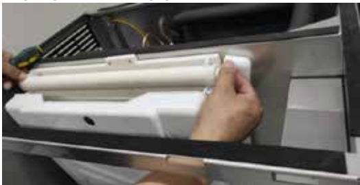
Unplug the water pipe
