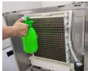
Flush the evaporator
