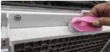
Brush the plastic parts around the evaporator
