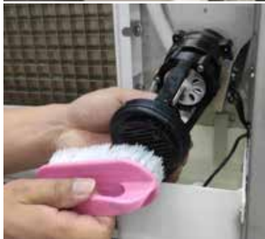
Water Pump Cleaning
