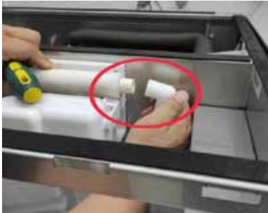
Unplug the water pipe
