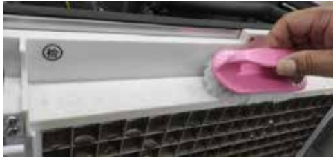
Brush the plastic parts around the evaporator
