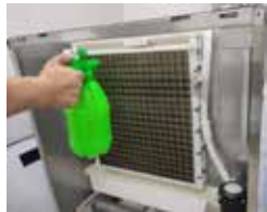
Flushing evaporator
