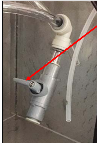
Fig. 2 Priming valve in OPEN position
