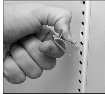
Fig. 1. Installing top tab of shelf clip.
