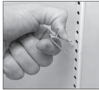
Fig. 1. Installing top tab of shelf clip.
