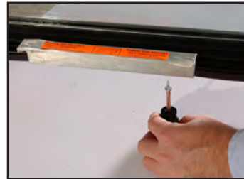
Fig. 2. Do not remove shipping brackets until unit is in final location.
