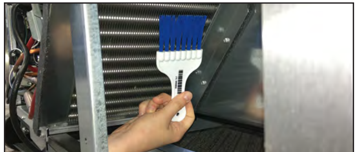
Fig. 3. Never brush across the coil fins.
