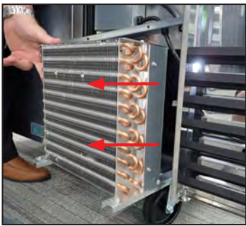
Fig. 6. Carefully slide the condensing unit out.
